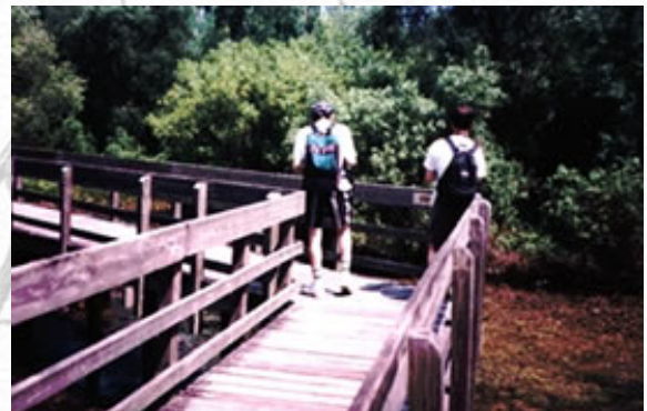
Elevated boardwalks for non-invasive observation of wildlife.
